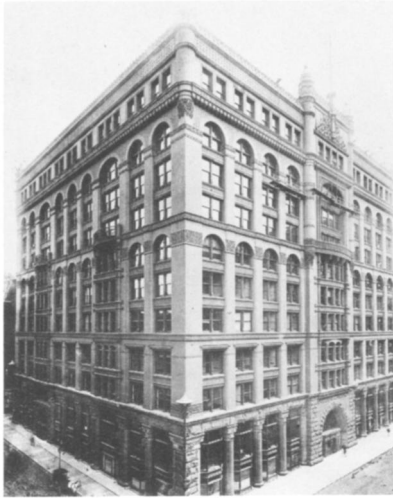
FIGURE 4. Burnham and Root. Rookery, 209 South LaSalle Street, Chicago, 1886–87. Considered the largest office building in Chicago at the time it was built, the Rookery was also acclaimed for its innovative central light court.
